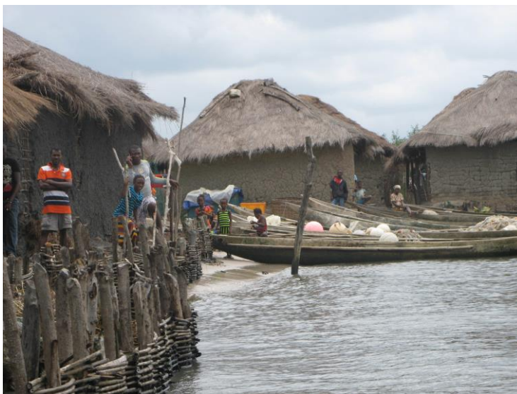
Figure E.1: General view of the village of Njajeiam. This view is typical of fishermen villages surveyed in this VA: dense build-up only few feet above the water level. Visible On the foreground are makeshift protections from the impacts of waves and storm surge. July 2016. Credit: S. Trzaska.
